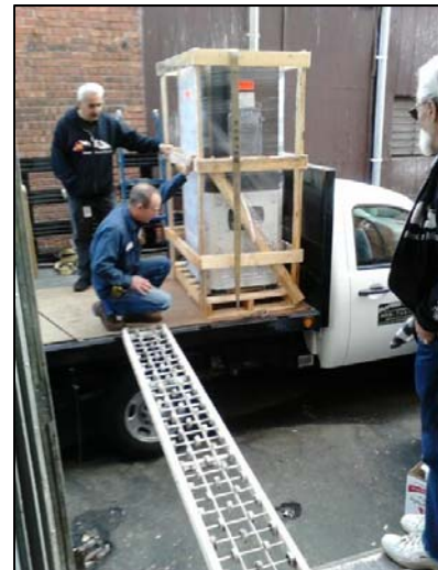
Domestic Hot Water Heaters are Delivered
