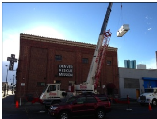
Dorm ERV is Hoisted to the Roof
