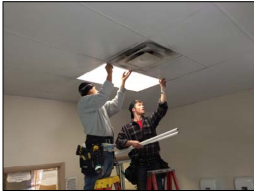
Lighting Upgrades in Progress
